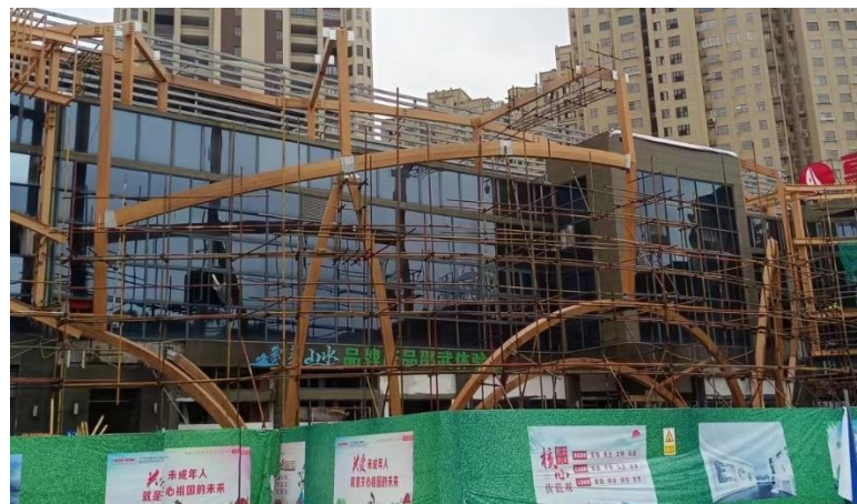
Fig. 18 Installation of bamboo members
