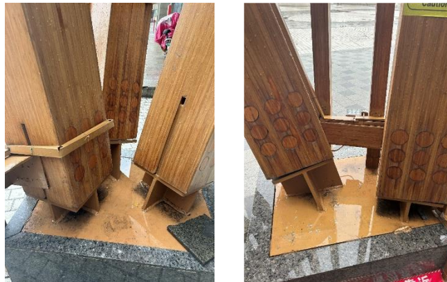
Fig. 7 Design of the LBL (bamboo) column base
