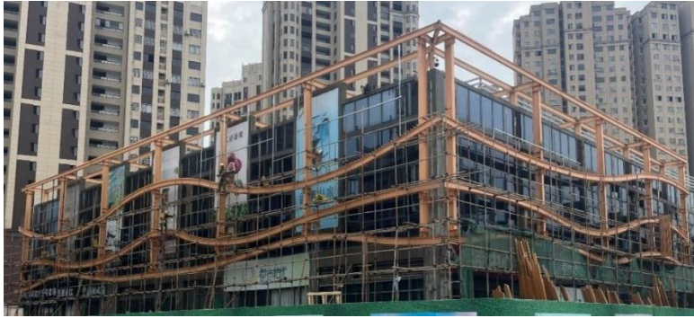
Fig. 9 Curved beams of the steel frame
