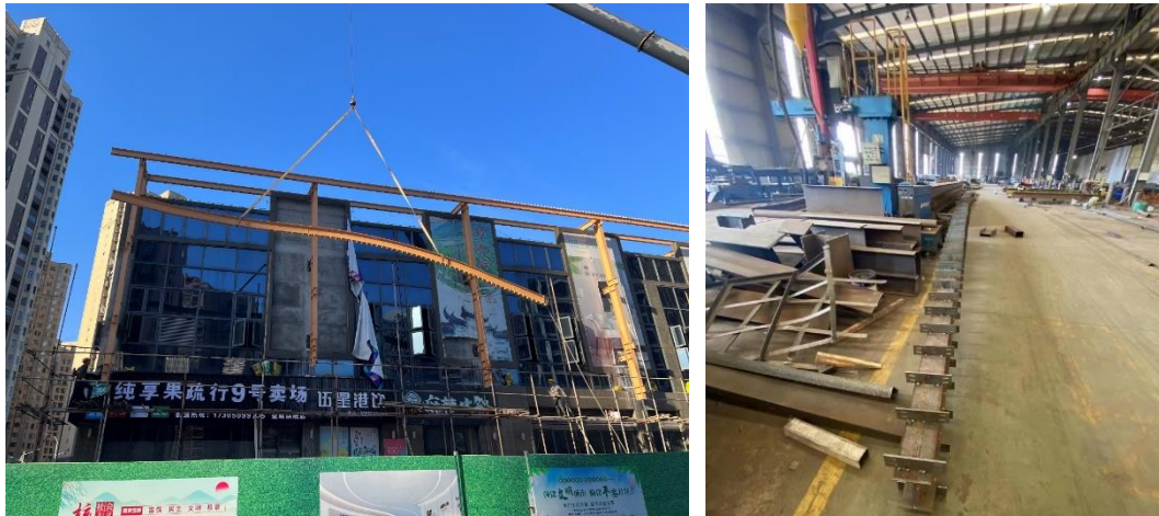
Fig. 13 Prefabrication and installation of the curved beam: (a) installation; (b) prefabrication.
