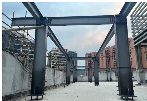
Fig. 12 Roof steel frame
