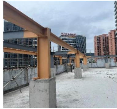
Fig. 10 Design of steel column base on the roof
