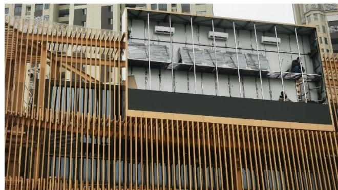
Fig. 15 Installation of the LED screen
