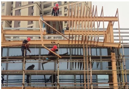
Fig. 14 Installation of bamboo grille
