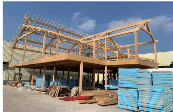
(h) Structural system for the whole building
