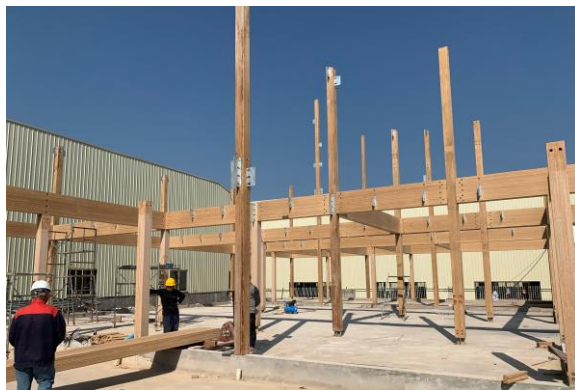
(g) Structural system for the first floor
