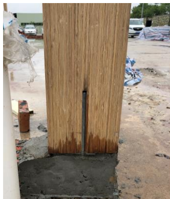
(e) Steel plate connection side
