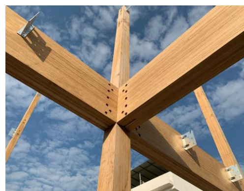
(f) Connections between columns and beams
