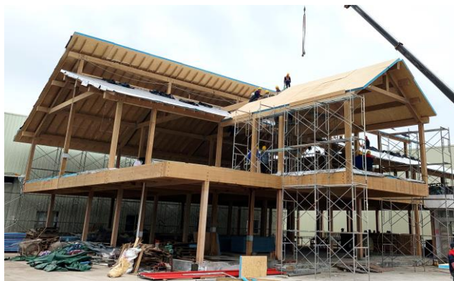
(i) Roof construction
