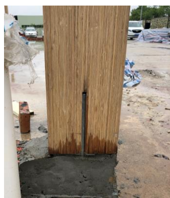
(e) Steel plate connection side
