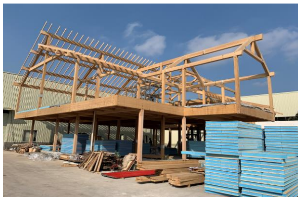
(h) Structural system for the whole building
