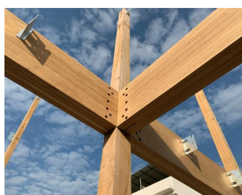
(f) Connections between columns and beams
