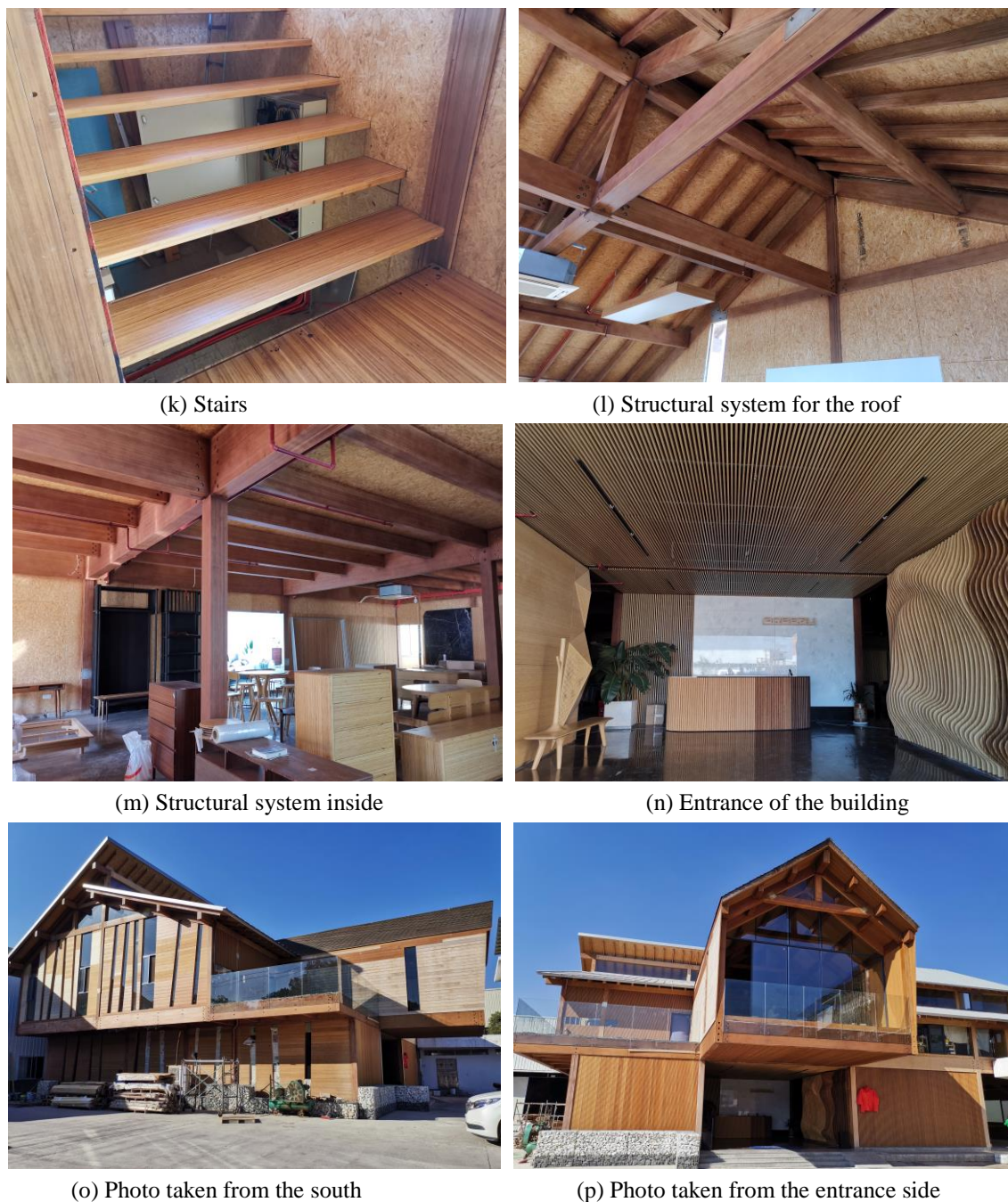
Fig. 5. LBL building construction
