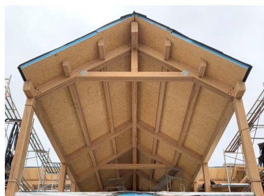
(j) Inner side of the roof
