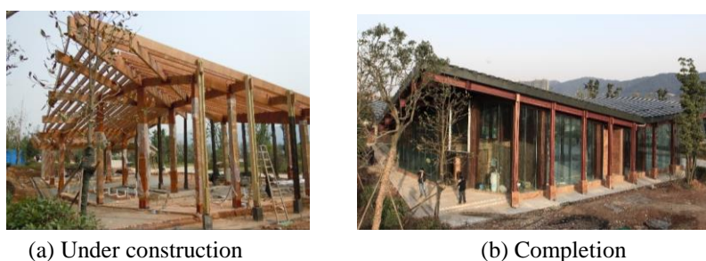
Fig. 2. Glubam beam-column structure building (Meixihu, Changsha).
