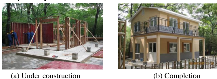
Fig. 1. Light glubam frame structure house (Zizhuyuan Park, Beijing).
