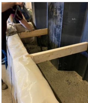
Fig. 12. Concrete poured around specimen.
