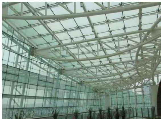
(b) Steel tubular truss at a theater in Henan Province, China
