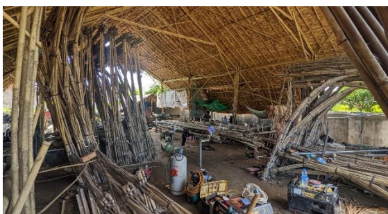
(a) Prefabricated bamboo trusses.
