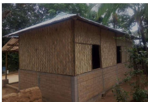
(a) Bamboo house under construction.
