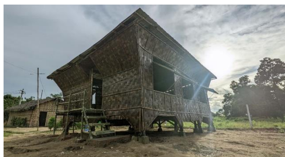
(b) Completed bamboo preschool.
