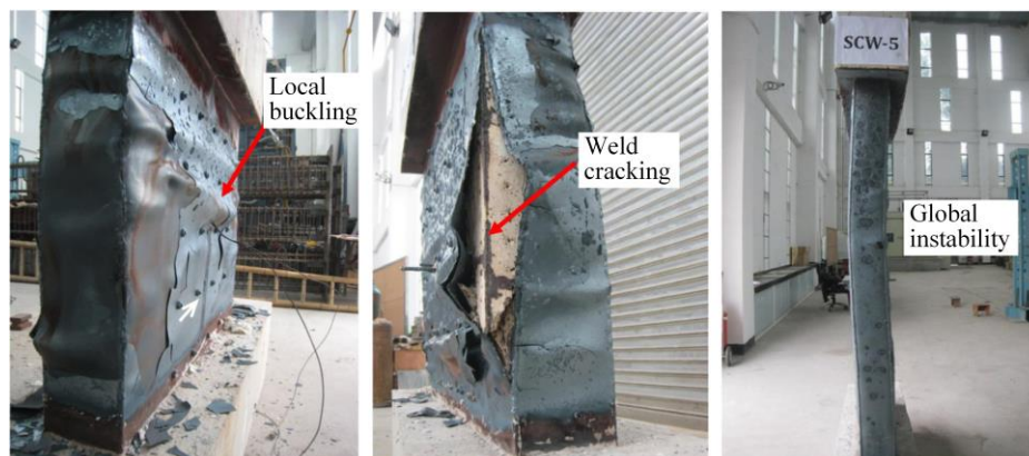
Fig. 14. Typical phenomena of DFPCW under fire exposure [78].
