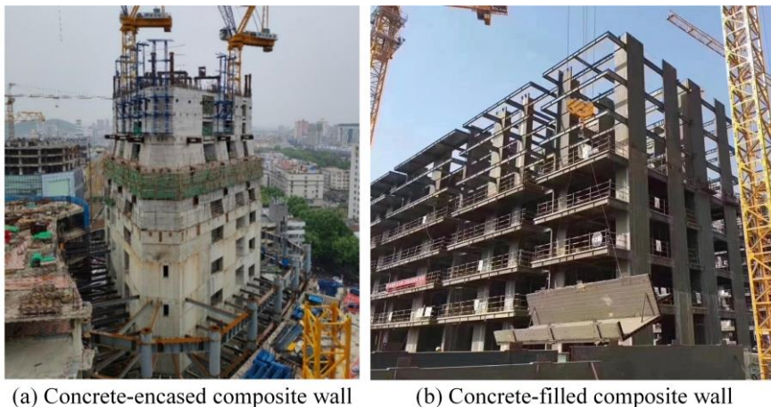
Fig. 1. Application of steel-concrete composite walls in practice [16, 17].
