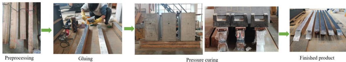
Fig. 4. Process of making FRP- bamboo scrimber composite beams
