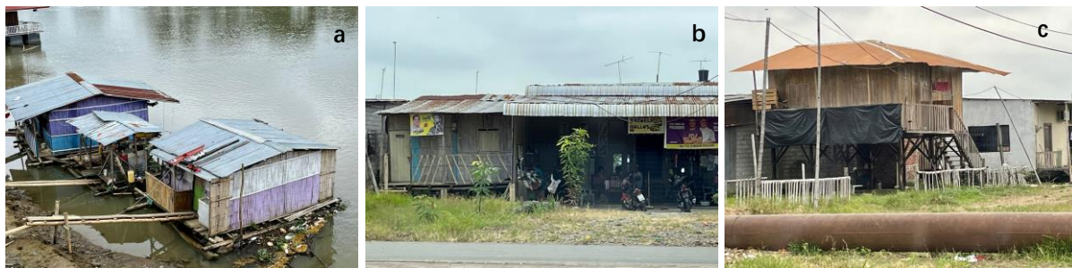
(a) Stilt houses with metal sheet roofing (b) Guadua cane houses (c) Guadua cane houses
