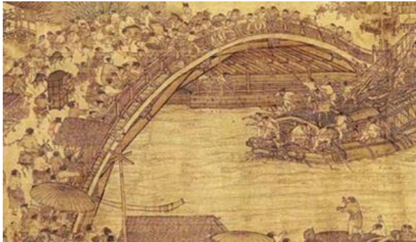
(a) Hong Bridge
