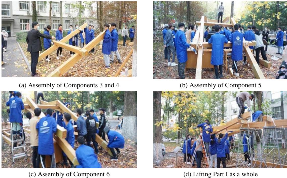
Fig. 14. Construction process of Parts I and III.
