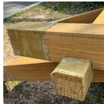
(b) GFRP wrapped near a connection joint
