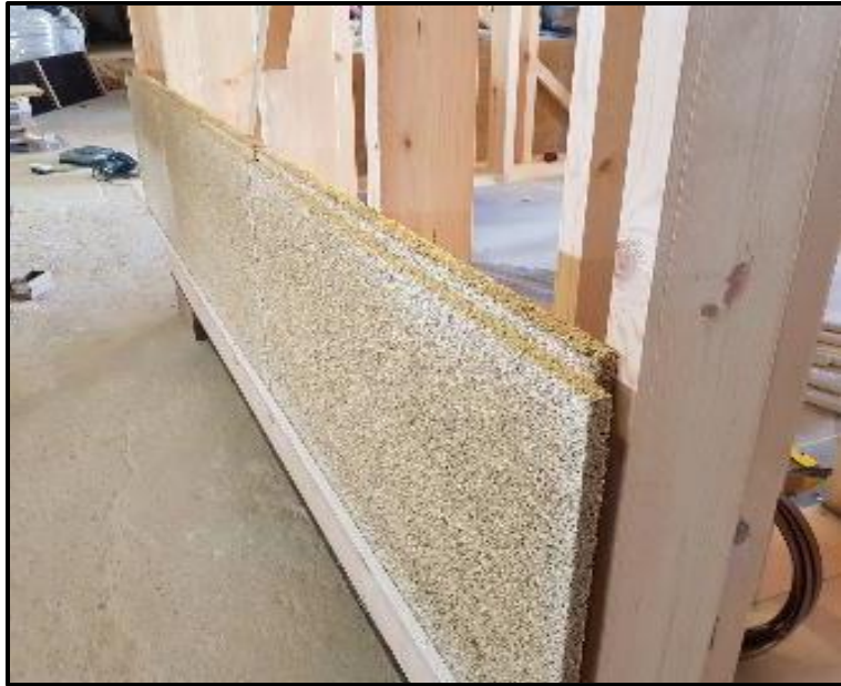
Fig. 6. Sandwich hemp concrete wall full-sized panel: dense MOC-hemp composite slabs on the outer sides; lightweight lime-hemp composite to be filled in internal layer (reproduced under the creative commons attribution license) [148]
