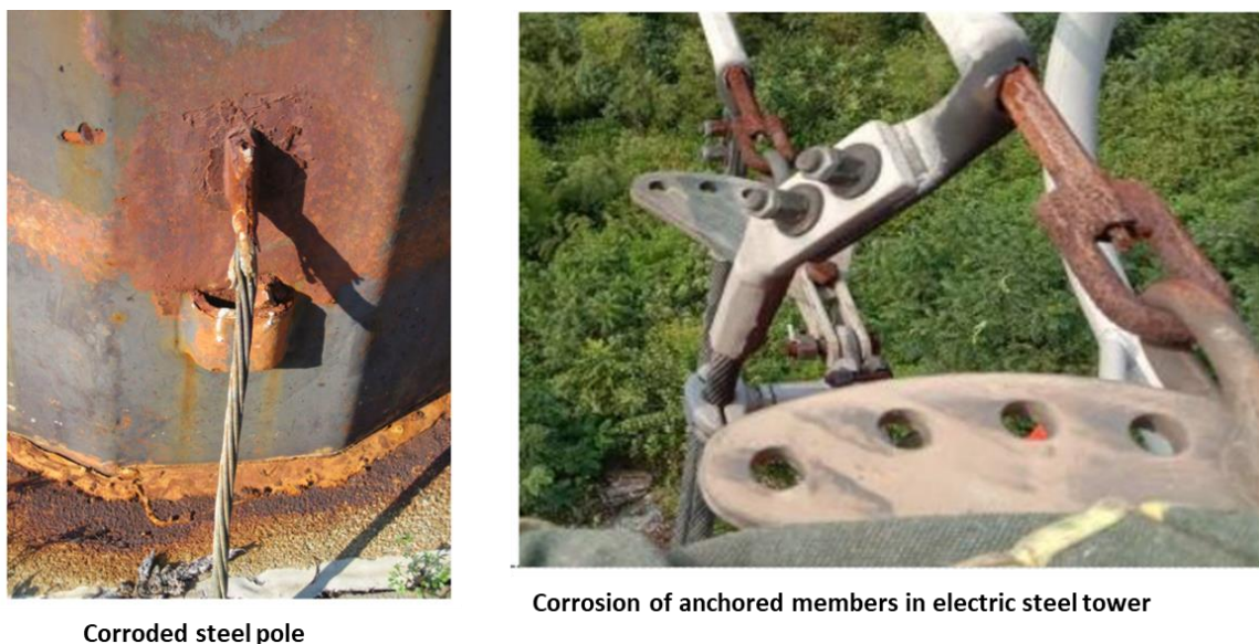
Fig. 7 Corroded steel poles and tower investigated [45,47].
