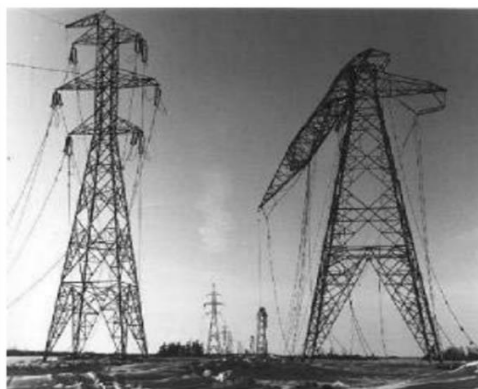
Broken Conductors and Tower Failure due to the 1998 Storm in Montreal
