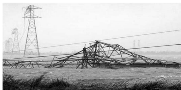
A Collapsed Power Pylon due to 1998 Storm
