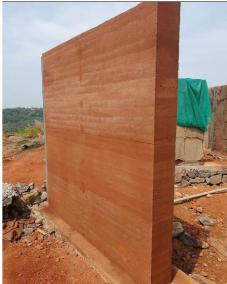
(a) Rammed earthen walls at a construction site, Calicut, Kerala, India
