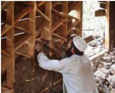
(c) A reconstruction program in the Pakistan-Kashmir region reviving the technique of Dhajji dewari, in which the small spaces between the timber studs are filled with stones and cob mixer [52]
