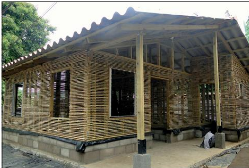
(a) Wattle structure of the bahareque construction made with a cane while constructing [27]
