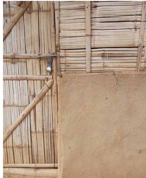
(b) Wattle and Daub walls built in Keystone Foundation, Kotagiri, Tamil Nadu, India
