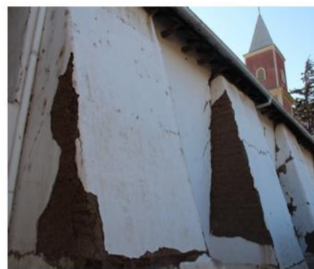
(d) An old church building of adobe construction provided with counterforts in Barraza, Chile [51]
