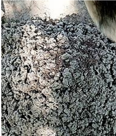
(a) Mixing of concrete
