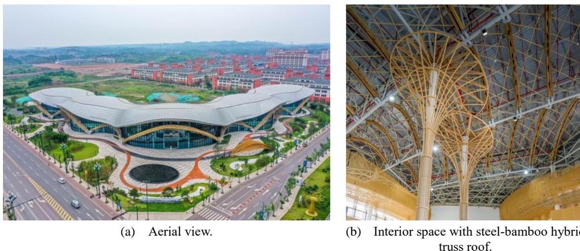
**Fig. 9.** Yibin International Bamboo Products Trading Centre. (Credit: Xi'an Construction Engineering Green Construction Group Co., Ltd)
