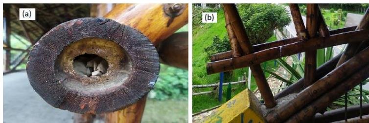
**Fig. 3.** (a) Section of *Guadua* elements, (b) Details of joints between elements.
