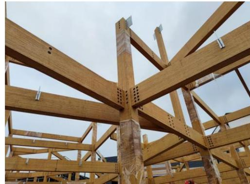
(b) Connection of beams and columns
