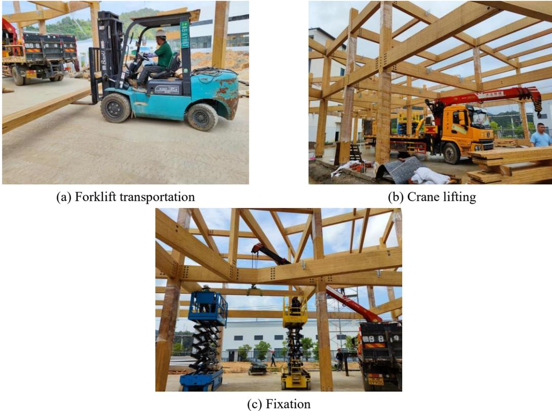
**Fig. 7.** Beam installation process
